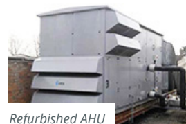
Refurbished AHU
