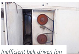
Inefficient belt driven fan
