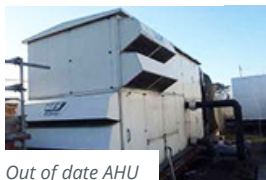
Out of date AHU
