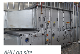
AHU on site
